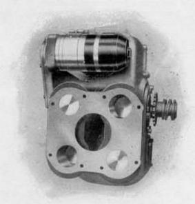
View showing how the twin crankshafts are geared together. Diagonally opposite pistons move in unison giving infinitely better balance than the conventional 4-cylinder in line car engine.
